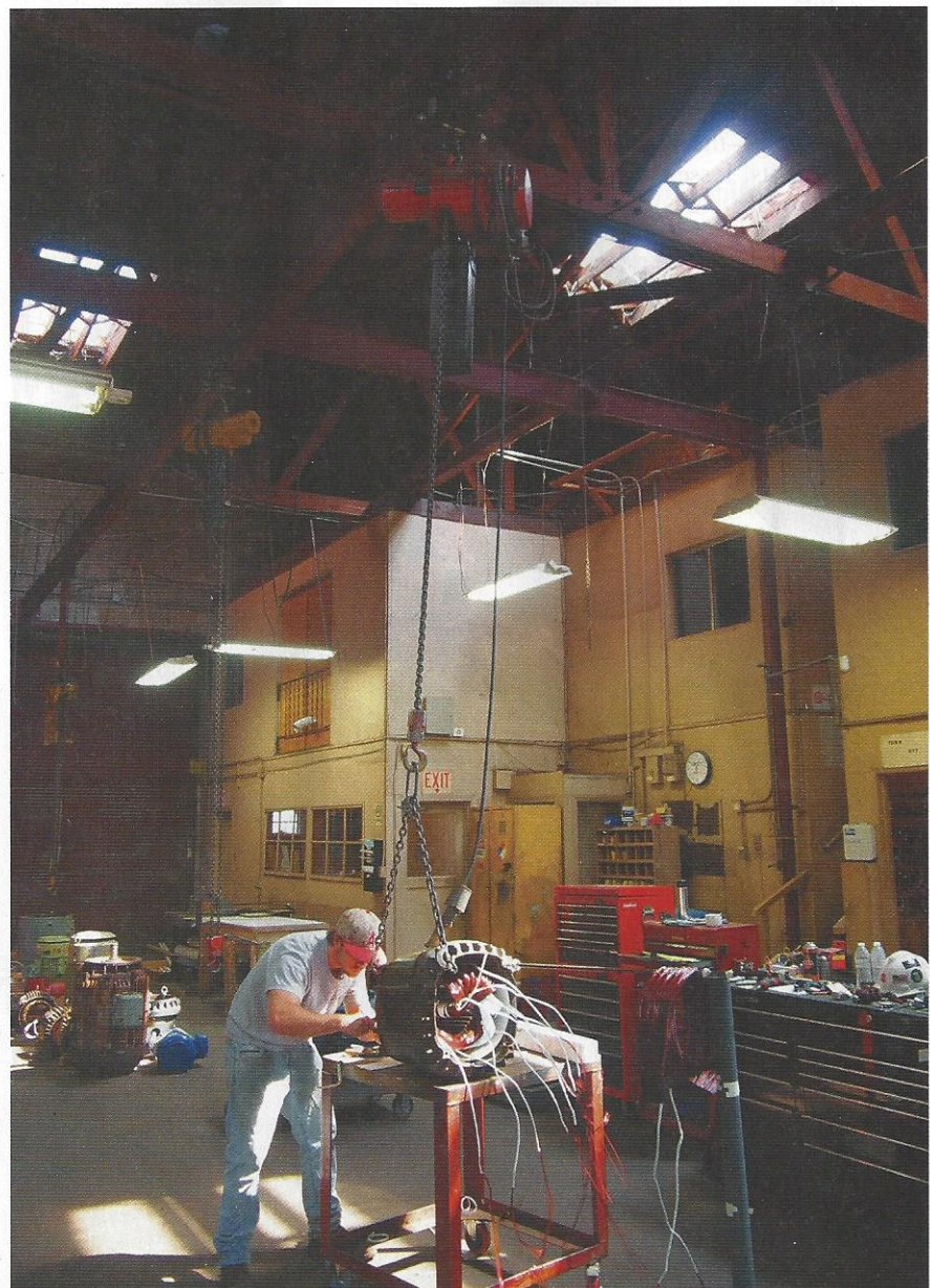
Vallejo currently uses a monorail crane but plans to install a bridge crane that will cover the entire facility and increase lifting capacity.
